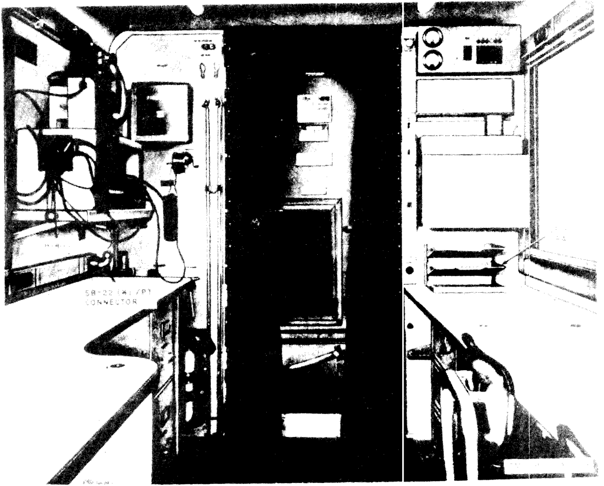
Figure 6. Operations Center, Communications AN/MS-31, interior rear view.
